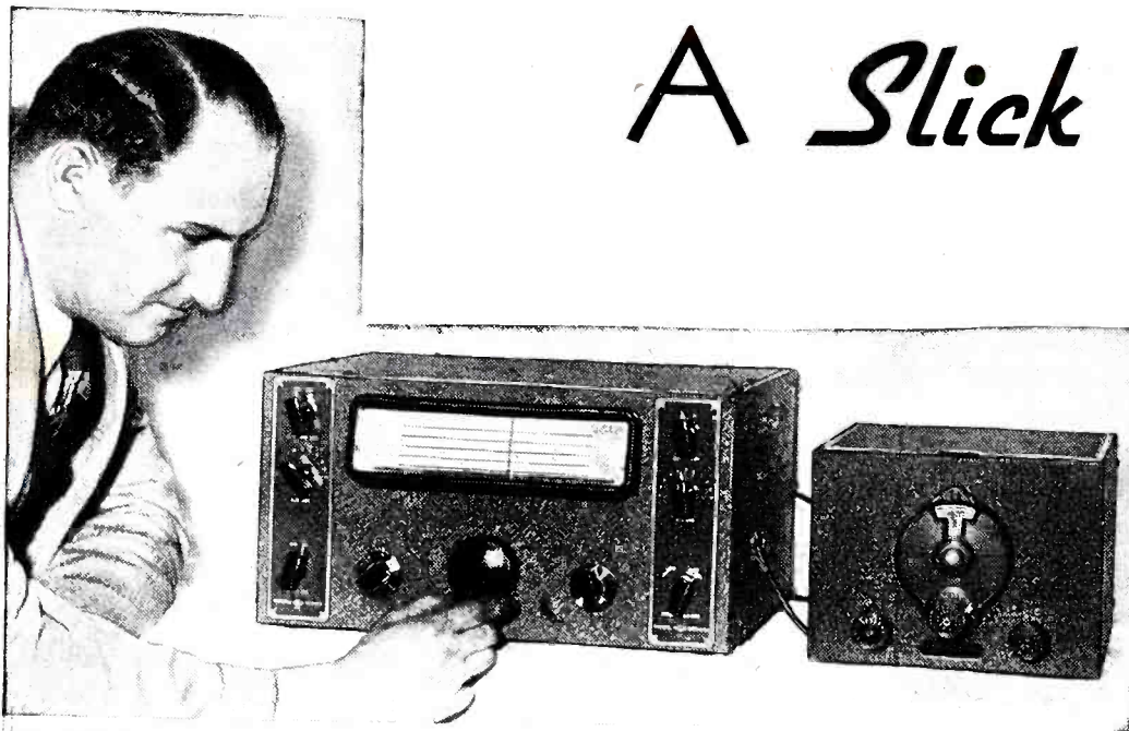
An SW-3 connected as a preselector ahead of a National NC81-X. Note the transmission line connected to the input terminals of the NC81-X.
